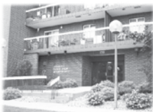
Jenkins Town View Apartments
